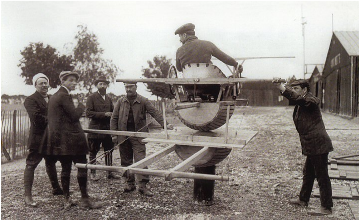
Figure 3.1: Synthetic flight training device (Moore, 2008)
